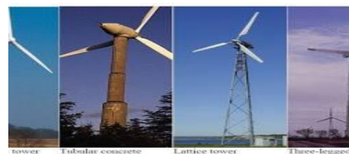
Fig: 1 Wind turbine tower
