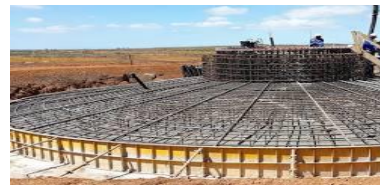
Fig: 8 Wind turbine foundation
