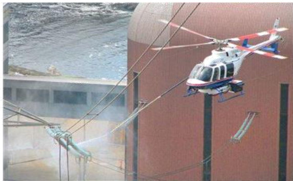
Fig 1. Hot line washing of insulators
