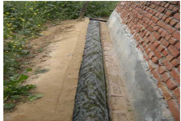
Fig.5. Drain out waste water
