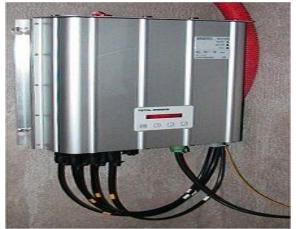
Inverter for grid connected PV Example of large 3-phase inverter for commercial and utility scale grid-tied PV systems
