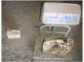
Weight batching of water and Admixture
